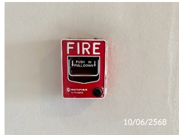
Fire Alarm Manual Station
